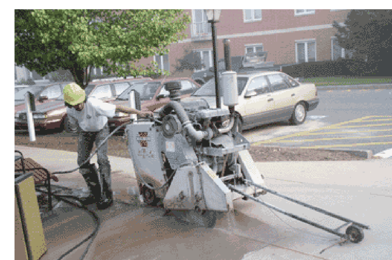
Figure 3. Example of silica exposure reduction method: concrete cutting with water.
