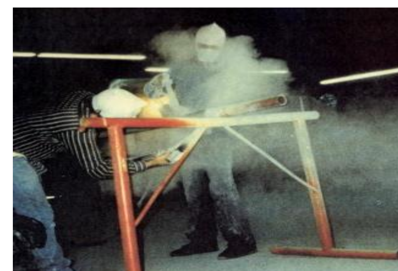
Figure 3. Example of silica exposure reduction method: concrete cutting with water.
